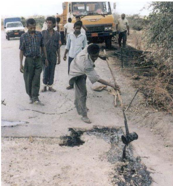
**Figure 4:** Rudimentary patching in Madagascar in 1997. When routine maintenance budgets are grossly insufficient, for traffic levels that are generally less than low, you cannot expect a complex and expensive network monitoring mechanism to last.
