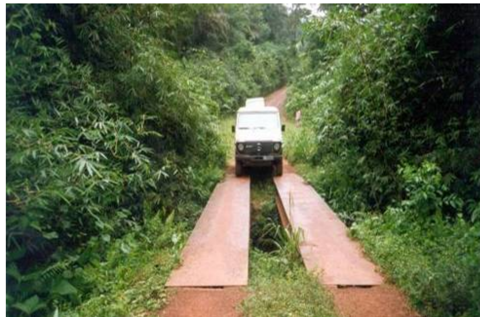
Bailey Bridge system for Rural Roads in Kindu / East Congo (GTZ Project) (Two double T-steel beams covered by iron plate for each lane)
