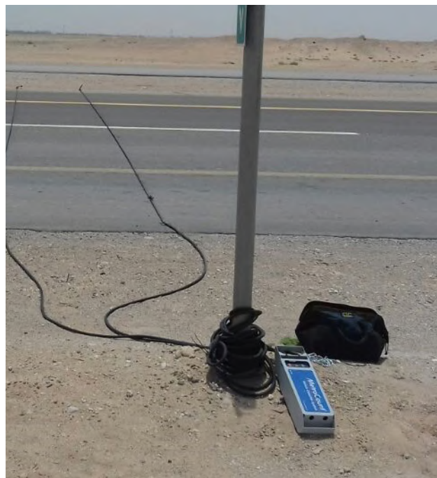
Typical instalment of pneumatic tubes for ATC.
