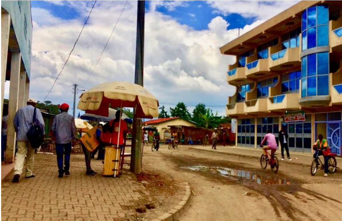
Figure 14: Roadway and NMT facility improvement needed in some parts of Musanze
