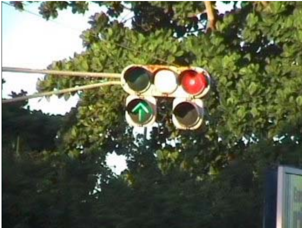
Fig. 6 Signals with right filter phase
