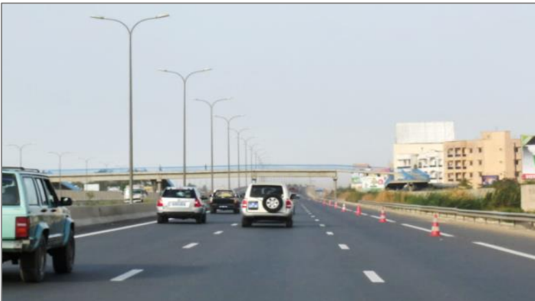
Figure 8 Dakar-Diamniadio Toll Highway – West of Pikine, Dakar
