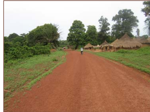
A newly rehabilitated gravel road in CAR
