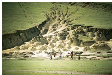
Caution is required in undertaking drainage work as interference with the natural drainage pattern can lead to major environmental damage in sensitive areas.
