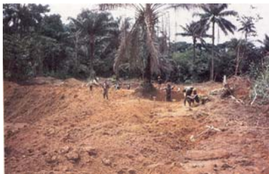
As-dug, nodular laterite gravel used in LVSR construction.
