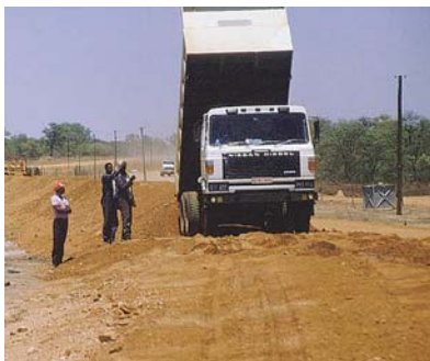
Breaking down of any oversize fraction will benefit the grading and quality of the available material.
