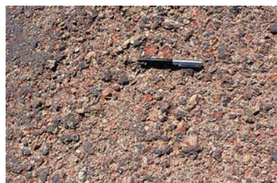
Example of a double Otta seal (using decomposed granite) after 10 years in service in a harsh, semi-arid environment with practically no maintenance.
