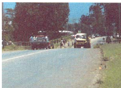
Poor visibility due to hidden sag curve - a potential cause of accidents.
