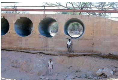
When there is a risk of erosion at outlets, suitable aprons and other protective measures are required.
