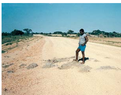
Burrowing animals such as termites can cause damage to pavement layers unless nests are removed properly and poisoned with an approved pesticide during clearing and grubbing.
