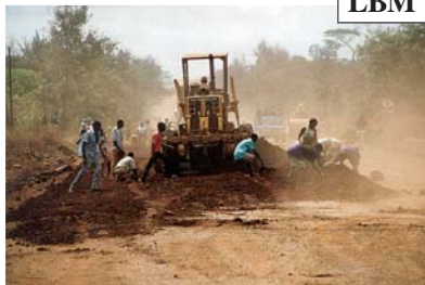
In most cases, the removal of oversize material is best carried out by the use of manual labour.
