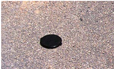
Sand seal surfacing.
