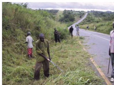
Grass cutting - a typical, labour-based, routine maintenance activity.
