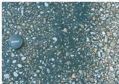
Single Otta seal with sand seal cover.
