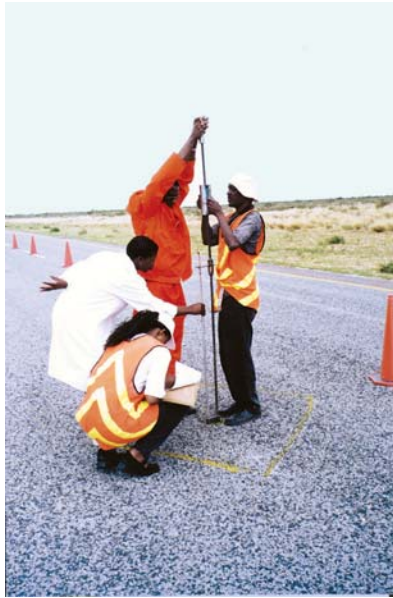
The DCP test in progress.
