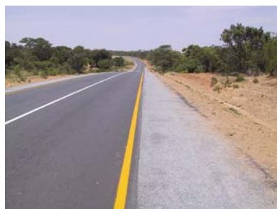
Figure 6.6 - Construction of sealed shoulders to existing bitumenised roads initially having unsealed shoulders
