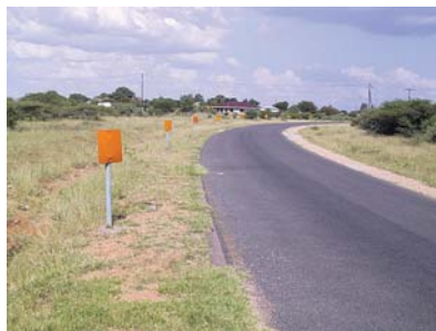
Additional signage should be provided on dangerous curves.
