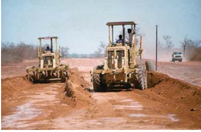
Graders are versatile for processing materials on the road.
