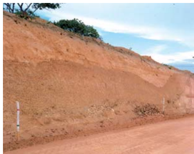
Laterite is a typical example of a “non-standard” material that has been successfully used in LVSR construction despite its non-compliance with traditional strength, grading and plasticity requirements.
