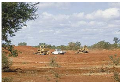
Reinstatement operations in a borrow pit.
