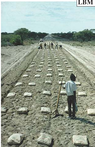
Stabilisation with lime or cement can be successfully applied with basic methods and use of manual labour.
