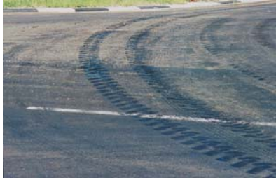
Heavy braking and tight cornering situations require an appropriate choice of high stability surfacings. Asphaltic concrete and possibly Cape or double Otta seals are preferred to sand, slurry, chip or single Otta seals.
