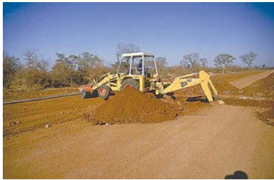
Excavators are convenient for various applications, including lifting.
