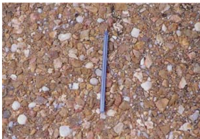
Screened gravel used as surfacing aggregate in the Otta seal.
