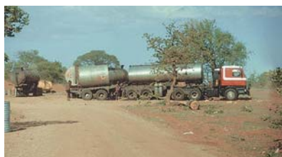
Handling of bitumen is a hazard and requires suitable locations for storage, heating or blending.
