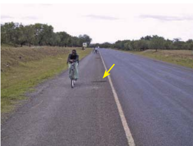
By deterring drivers from using road shoulders, the use of shoulder humps can improve the safety of pedestrians and cyclists
