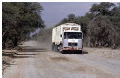
Road upgrading requires careful planning to minimise adverse impacts on the natural environment.
