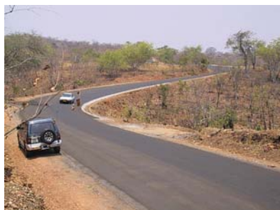
Good combination of curves and adequate horizontal curvature provide for a safe road environment. However, a lack of road markings constitutes a serious safety hazard.
