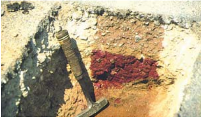
Phenolphthalein reaction in stabilised sub-base.
