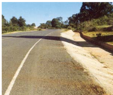
Good sight distances on a well-designed LVSR. Note wide shoulder and shallow slope to drainage ditch which both reduce potential hazards.
