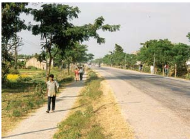
A segregated footpath can be a cost-effective means of catering for high volumes of pedestrian traffic.
