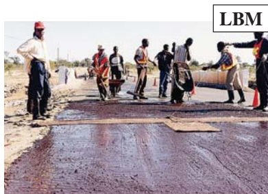
The slurry seal lends itself to construction by labour-based methods.
