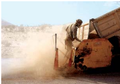
High contents of dust and fines in the aggregate are more critical for the good performance of a surface dressing than for that of an Otta seal.
