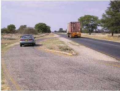
Lay-bys provide a safe haven where vehicles can pull off the road.
