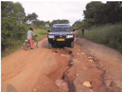
The bulk of the SADC rural road network is still unsurfaced and in relatively poor condition.
