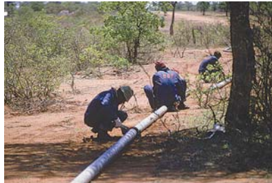
Supply of construction water may involve the construction of temporary pipelines.
