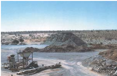
(a) Original pit used for construction.
