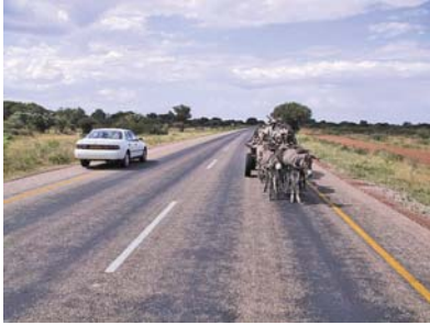
Shoulder sealing is highly beneficial to the performance of LVSRs, especially where moisture sensitive materials are used.
