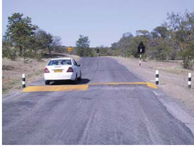
Well-designed speed humps are an effective means of slowing down traffic.
