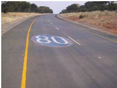
Speed limit painted on the road.
