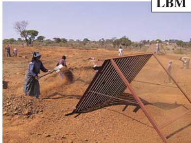
Screening aggregate by labour-based methods (Otta seal is shown, sand seals would be similar).
