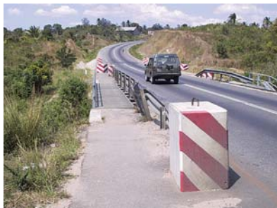
A segregated footway on a narrow bridge provides protection for pedestrians.
