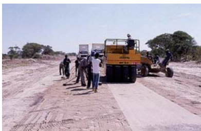
Rolling of sand seal.
