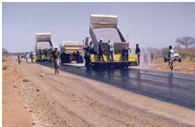
Applying aggregate for surface dressing using mechanical chip spreaders.
