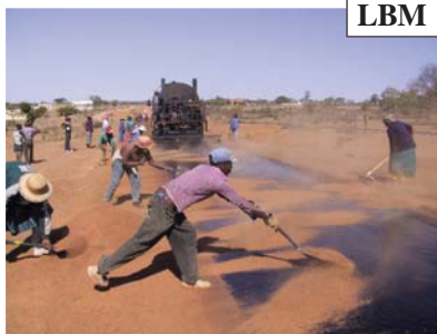
Spreading gravel using labour-based methods. (Otta seal), from heaps placed along the road.
