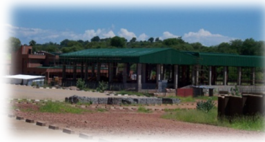
Chirundu commercial freight building under construction in Zambia
