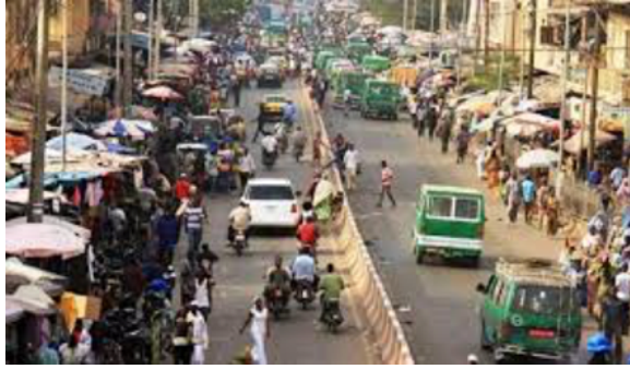
Figure 9 | Road infrastructure of the primary network, Sotrama Ring Road 25
