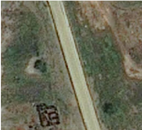
Good Condition (smooth texture, consistent width)
