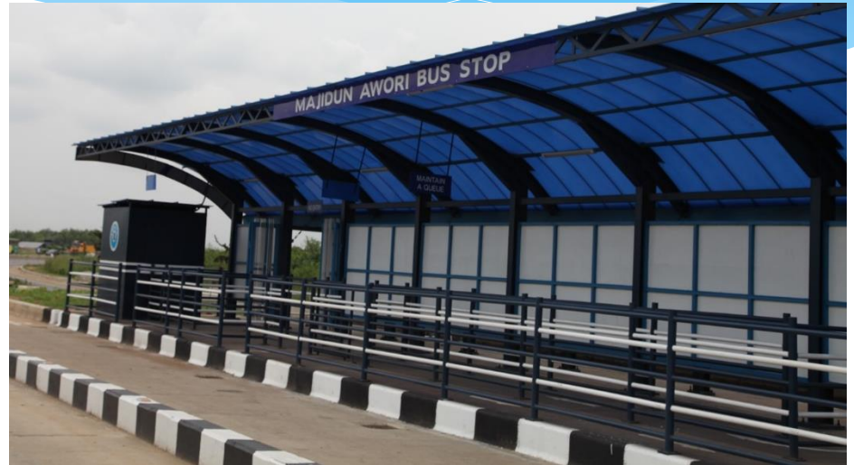
BRT Ext Bus Shelter
