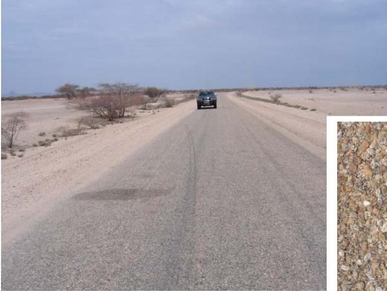
The double Otta seal surfacing constructed from screened quartzitic gravel obtained from adjacent to the road alignment.
