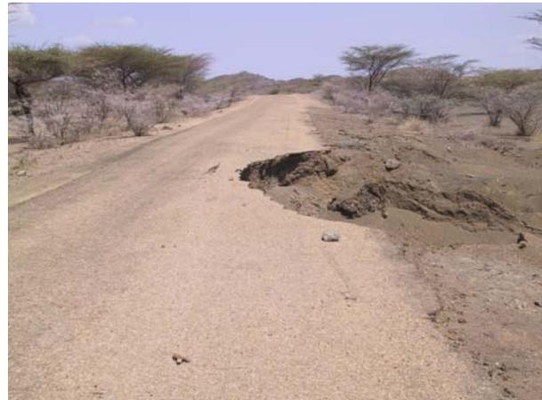
Examples of poorly designed drainage structures along the Marich Pass – Lodwar road. Insufficient depth of the downstream skirt has resulted in extensive scour of the drift (left) and a washout at a culvert outlet along the Lodwar-Kalokol road.
