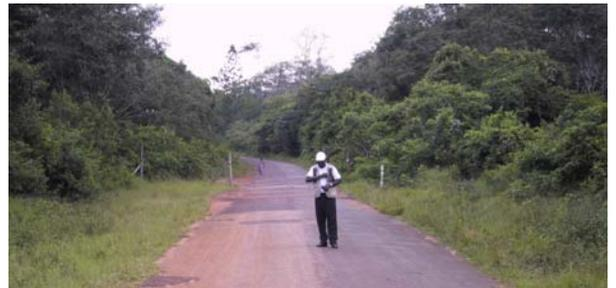
Kwale trial, "as dug" laterite as Otta Seal
