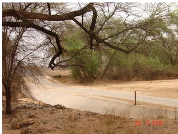
Examples of well designed drifts along the Marich Pass-Lodwar road in which the bottom of the drift, forming the road surface is exactly at the level of the river bed – a requirement for good performance.
