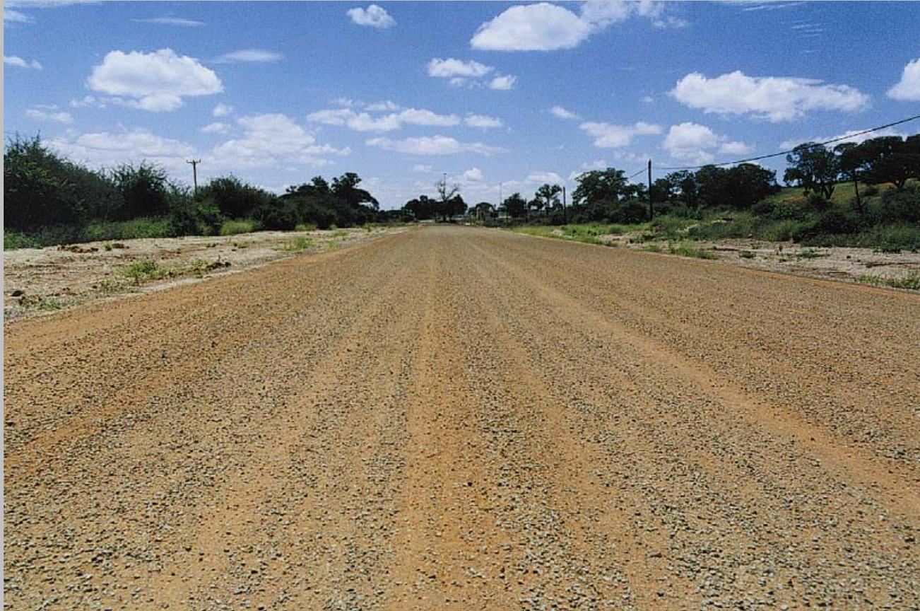
**3 - 4 weeks after Construction, some Excessive Aggregate has been Dislodged by Traffic**
