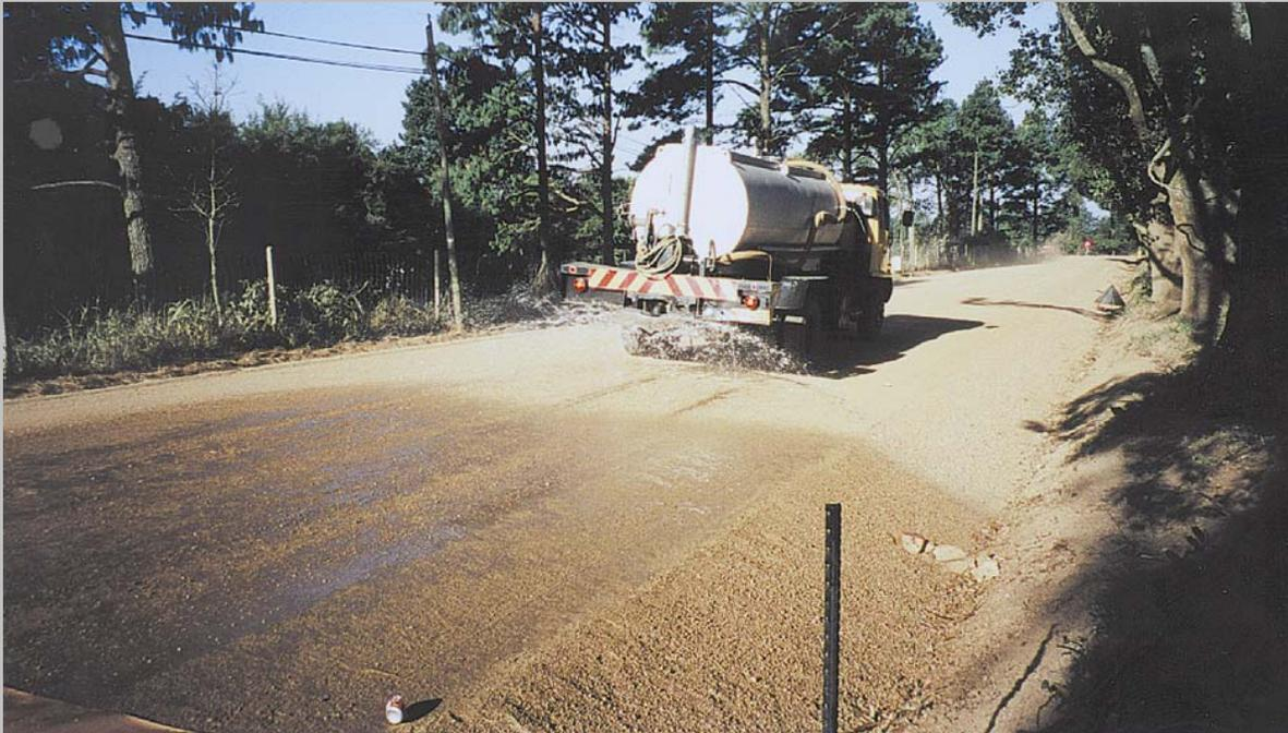
Light watering of the broomed base before spraying, the binder will enhance the bond between the surfacing and the base layer.
