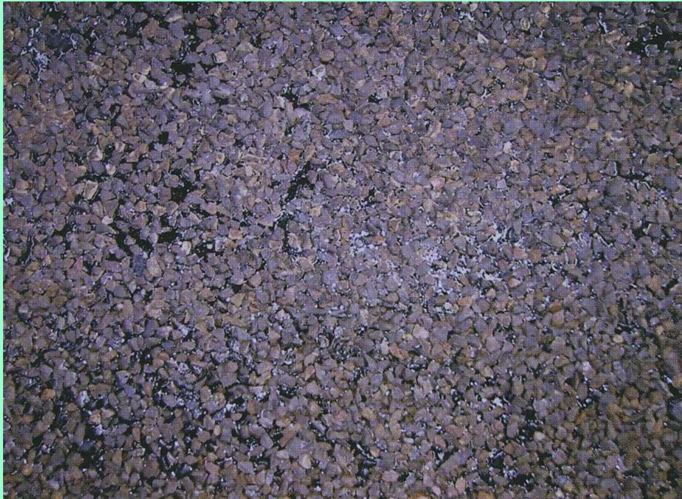
**Newly placed sprayed surfacing. Note the gap between the aggregates which allow the 2<sup>nd</sup> seal to mesh in.**
