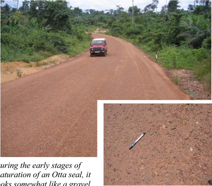
*During the early stages of maturation of an Otta seal, it looks somewhat like a gravel Road. However, after 6 – 8 months the surface takes on the appearance of asphaltic concrete*
