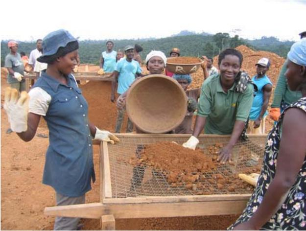
Oversize aggregate was removed by labour based methods with a good results. At a later stage a vibrating screen took over this work as seen below.
