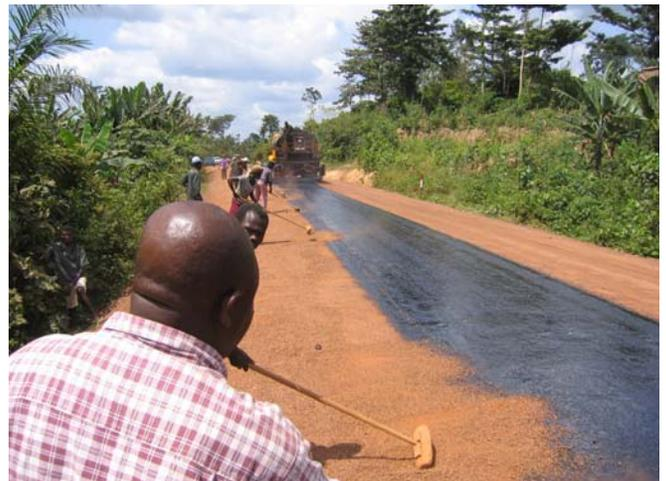
*Spraying of bitumen with the use labours brooming back aggregate for the longitudinal joint immediately spraying the bitumen.*
